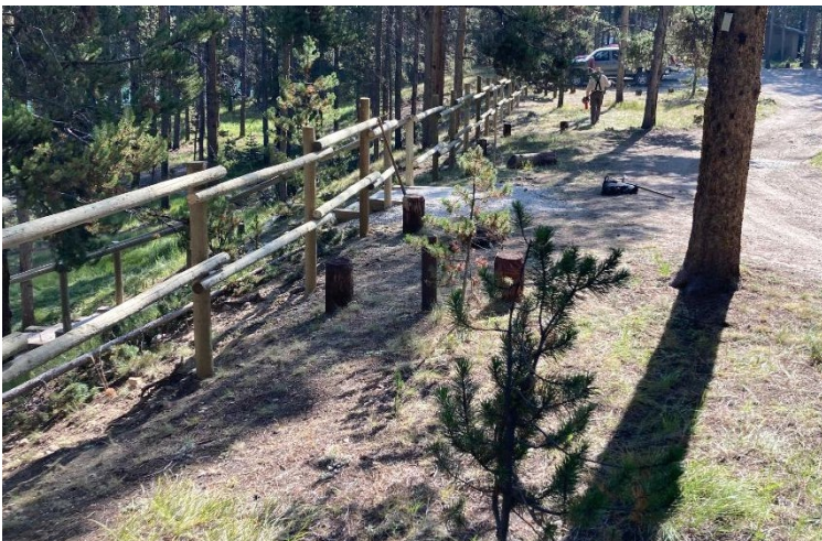
New fence and graveled trail in the refurbished campground.
